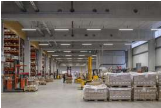
Fig. 4: Annual power consumption could be reduced from 1.2 million to less than 465,000 kilowatt hours. This means a reduction in CO 2 emissions related to lighting by almost 139 tonnes per year – amounting to just 38.6 per cent of the former level.
