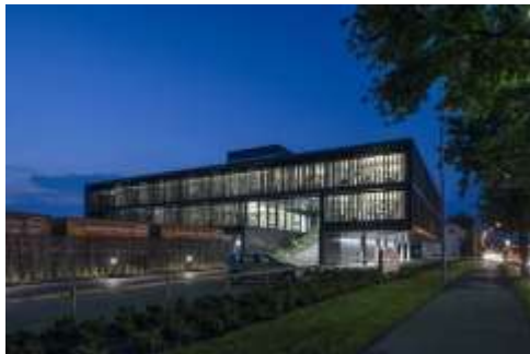
Fig. 1: Gebrüder Weiss, one of Europe's most important transport and logistics services providers based in Lauterach, Vorarlberg, continues its long-standing collaboration with Zumtobel.
