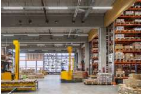
Fig. 2: Due to their high energy efficiency, LEDs have played a major role in building new and refurbishing existing buildings of the logistics hubs of Gebrüder Weiss in compliance with environmental considerations.
