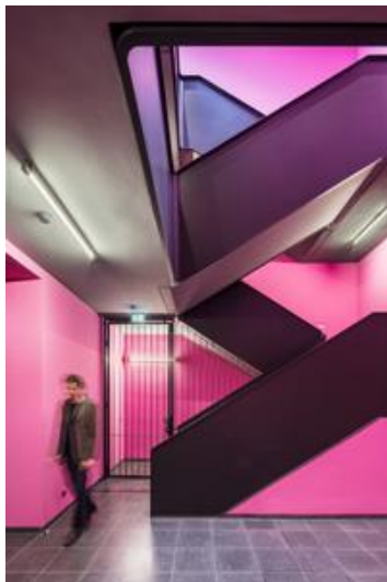
Fig. 3: Simple and slim Zumtobel LINARIA light lines in a customised black colour were chosen for the stairwell lighting, with an integrated emergency lighting connection.
